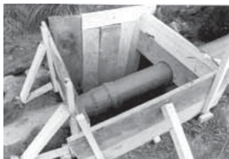
FIGURA 11: ANCLAJE DE TUBERÍA
